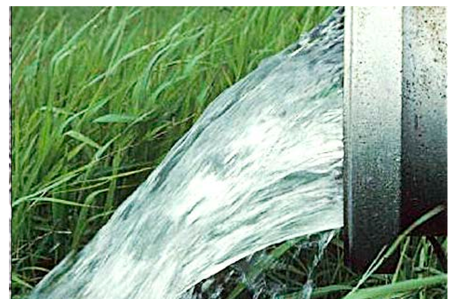
Electrowinning for waste water treatment.
